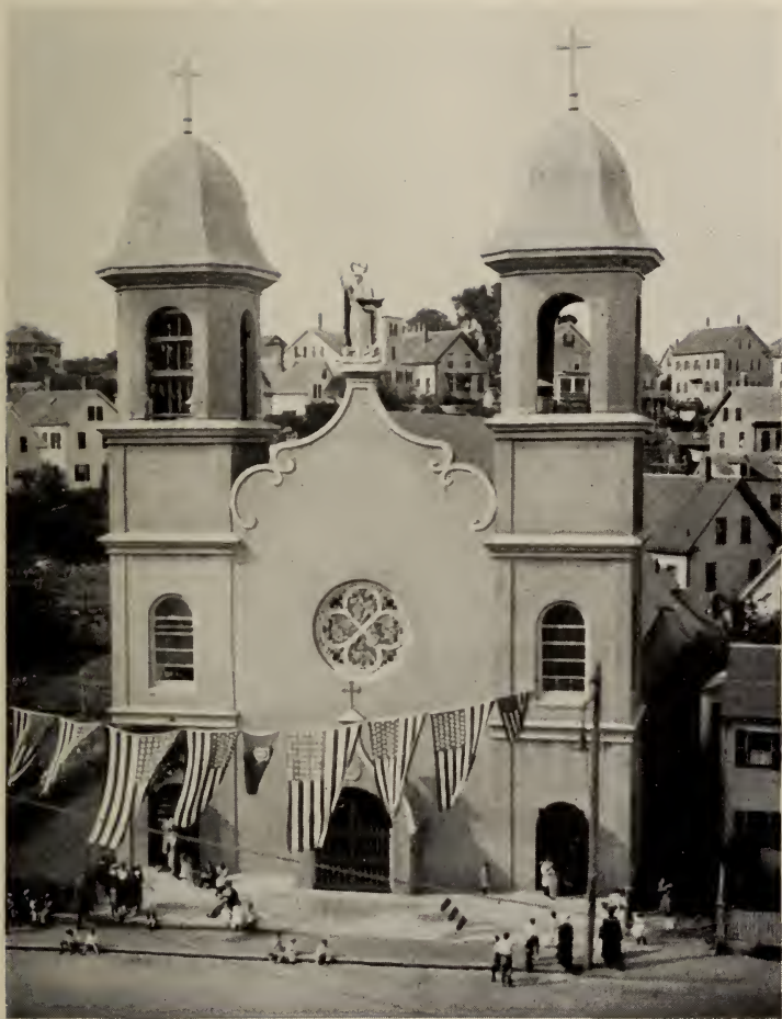
GLOUCESTER OUR LADY OF GOOD VOYAGE CARILLON TOWER
